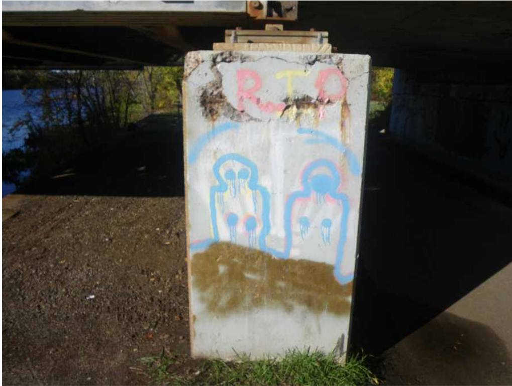
Photo 47: Pier 8, East Pedestal, East Face, Looking West - Full width spalled area with exposed rebar.
